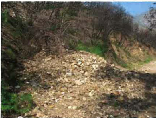
Erosion, due to lack of brush, poses a flood risk.
